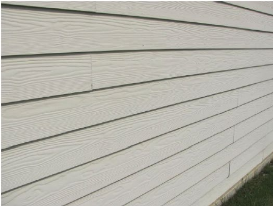
Fiber cement siding
